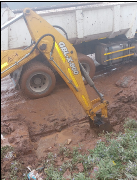
STORM WATER DRAINS CLEARED
